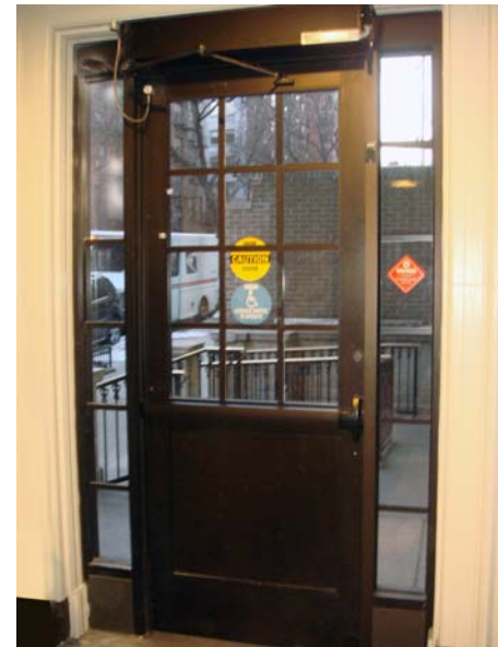
Exit device can be retrofit to a wide variety of door types and can be used with automatic openers
