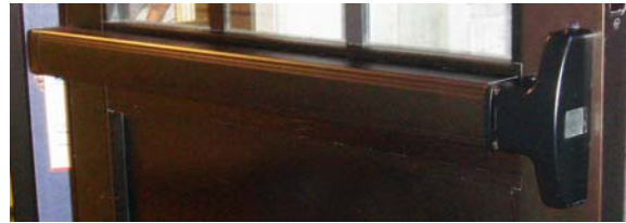
Exit device shown with latch electrically held-back
