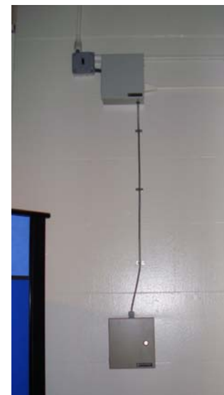
Power Supply & Timer Supplied connected via armored cable for easy installation
